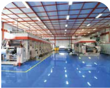
Industrial Flooring Solutions
